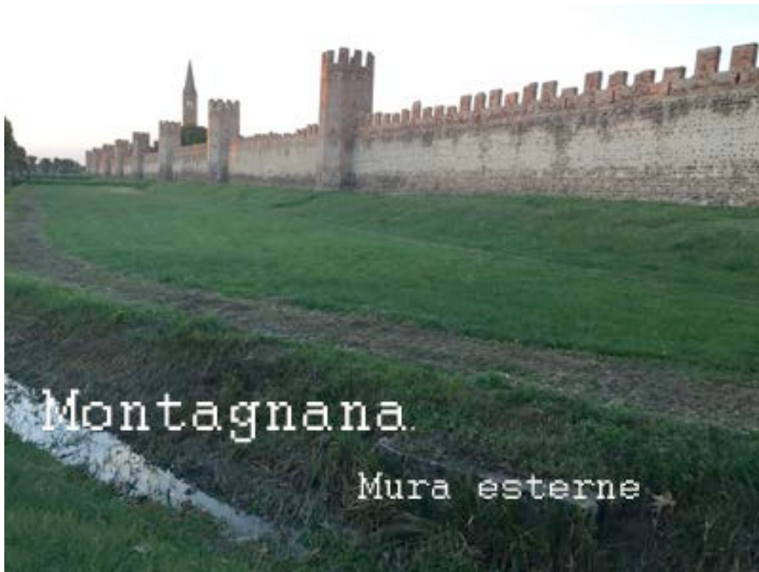
The wall outside
